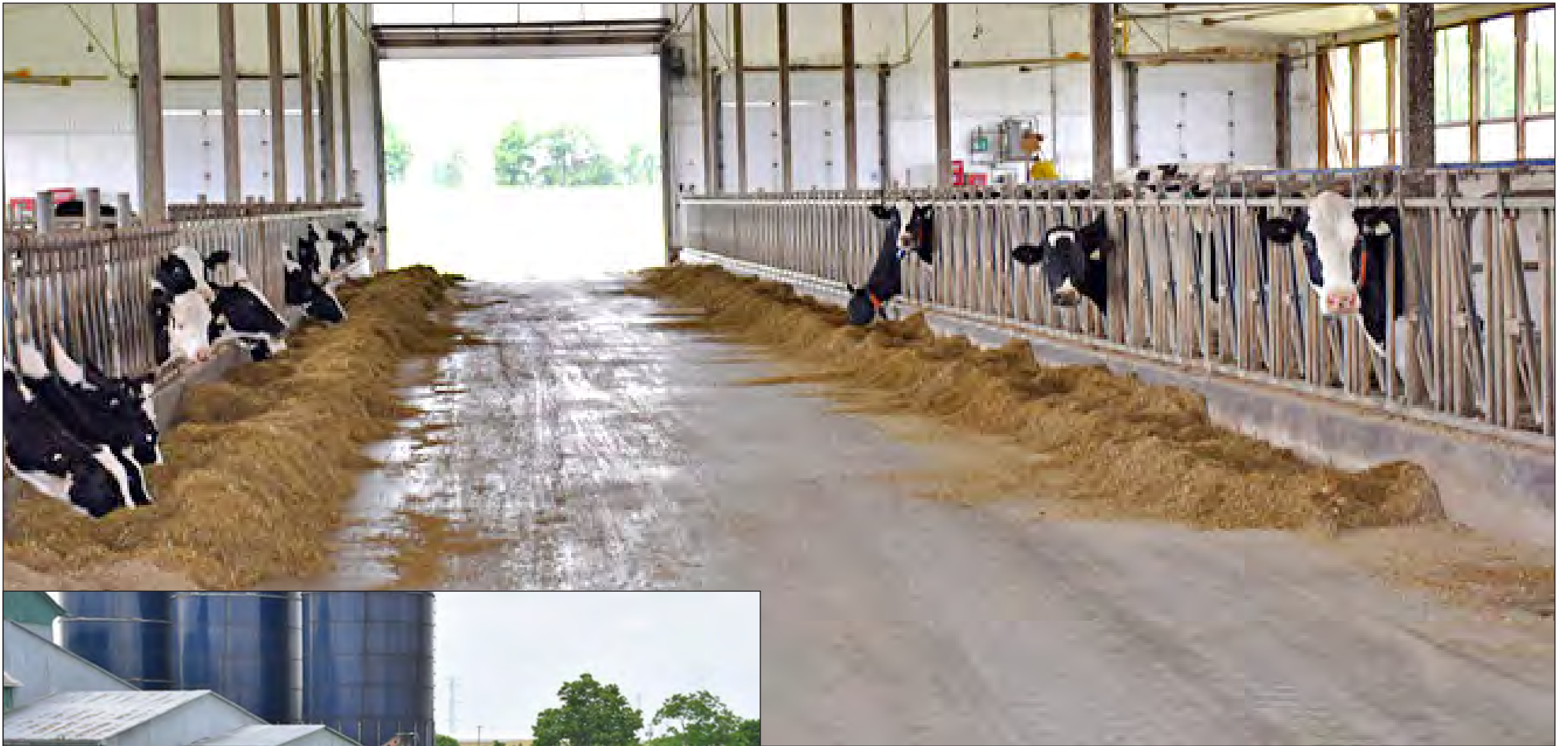
A view of the new barn at Posslea Farm.
